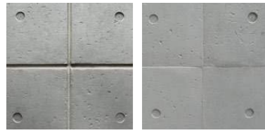
10 mm Grouting No Grouting
