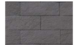
BK-1206 without grouting
